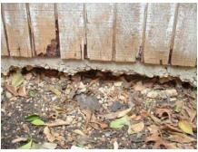
The rear addition is visibly separating from the main structure.
