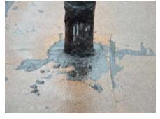
Active roof leakage was observed at the right rear side of the structure at the roof overhang (see the exterior walls section).
