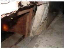
The exterior walls/siding exhibit very poor protection against the elements at various siding and trim junctures and at exterior wall penetration points, and there are many areas were wood surfaces are exposed to damage. A thorough reevaluation of the exterior siding's ability to shed water and prevent water penetration is recommended. Also, see further below.
