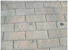
There are several areas visible where repairs have been made to the roof surfaces with a considerable amount of sealing tar. It could not be determined how effectively these repairs were made.
