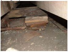
Crawl space portions of the structure do not have adequate crawl space ventilation.
