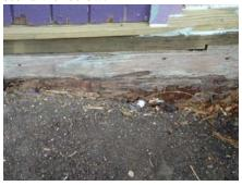
Some areas of composition type siding are quite water damaged, such as near the main electrical meter.
