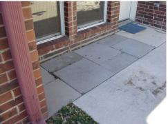
Roof runoff exists (poorly functioning or non-existent gutter system). The right side of the home does not have a gutter system.
