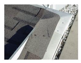
There are area of the roof or roof components that have been patched with an excessive amount of sealing tar. (patches of this type are temporary in nature and generally require ongoing maintenance).
