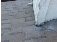
Poor seal noted at various exterior wall penetration points (i.e. Freon line entry point, exterior light fixtures, exterior faucets, etc.).
