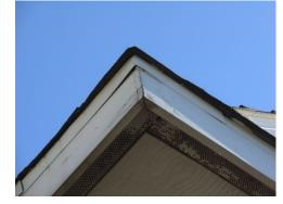
Fascia boards are separating at joints and/or are twisted/warped.
