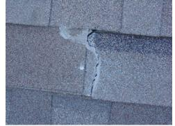
Exposed and improperly sealed nail and/or staple heads are visible through the shingle surfaces and/or flashing areas.
