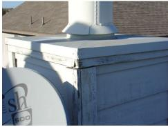
The siding and/or trim is in direct contact with the roofing material(s) at the chimney.
