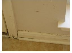
The baseboard(s) is water damaged in the master bathroom adjacent to the shower stall and hall bathroom adjacent to the bath tub. Both areas are a result of water splash out from the adjacent shower and bath.
