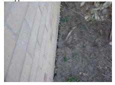
Soil erosion exists adjacent to the structure in several areas. There is not positive drainage away from the foundations in many areas as a result.
