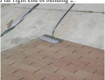
Some shingles are scuffed/damaged, apparently from previous branch contact. Examples are visible at the front center of building 1 and at the left front of building 3.
