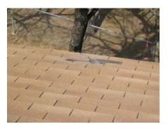
There are exposed nail heads visible at many of the vent pipe flashings, where shingles have been pinned, and also at building 1 there are many exposed nail heads near the ridge vents.
