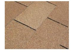
Shingles are torn or have blown off of the roof surfaces at all three of the buildings. It is recommended that these items be repaired immediately. There are roughly half a dozen to a dozen damaged shingles on each building.
